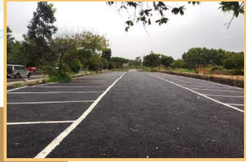
Development of Parking area
